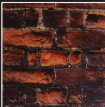
RESTORATION & REPAIR WORK
